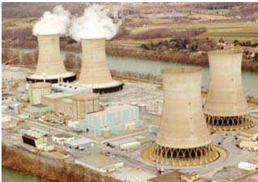
Nuclear Power Station
