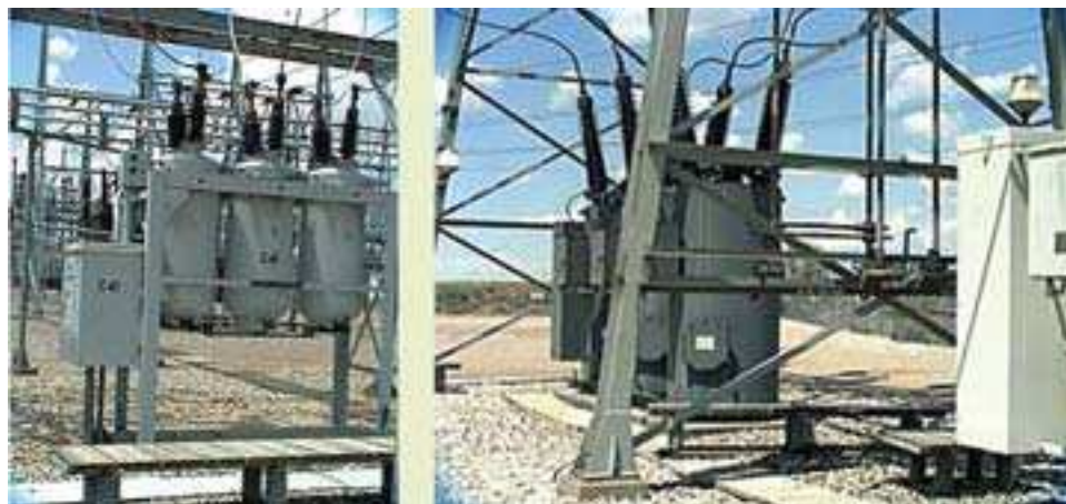
Oil Circuit Breakers
